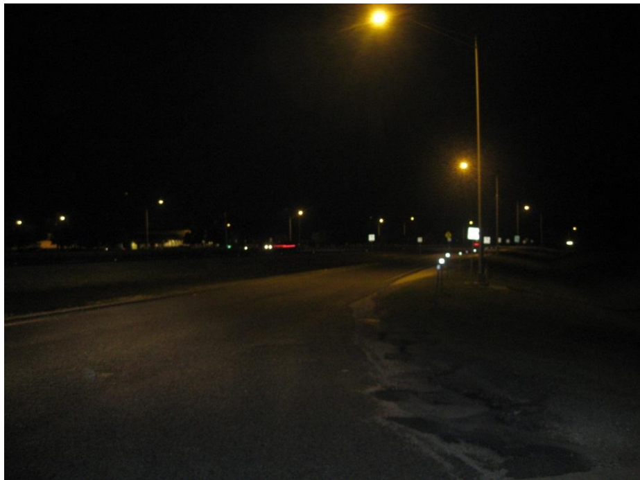
Figure 28: Ruined pavement due to shoulder parking at St. Johns
