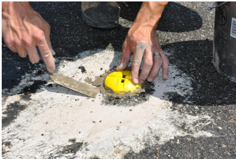
Figure 41: Sensor being installed by the technician
