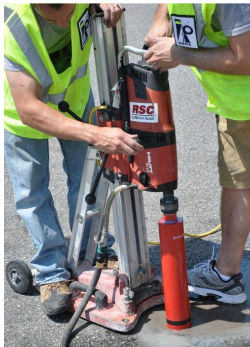
Figure 38: Core drilling process
