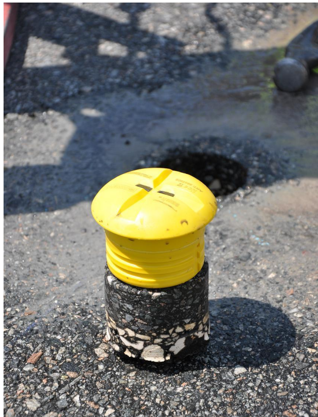
Figure 40: The removed core and the sensor to be installed
