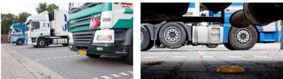
Figure 30: Wireless vehicle detection system application at a rest area in Europe (Source: www.nedapavi.com )
