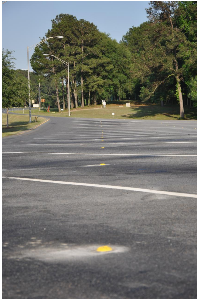
Figure 42: The first row of sensors after installation
