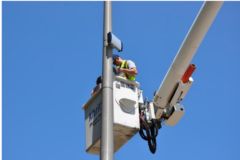
Figure 45: Data collector mounted to light pole
